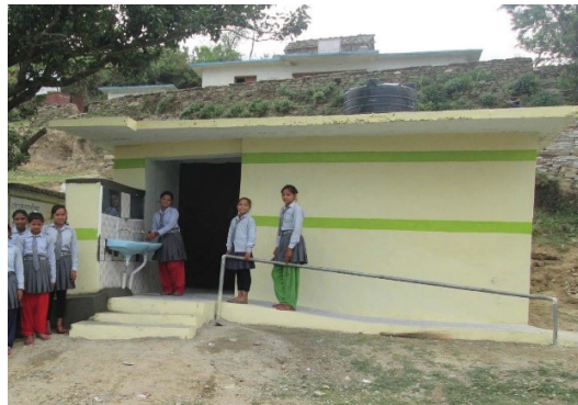
Fig. 5. Menstrual hygiene management-friendly toilet, Doti district.
